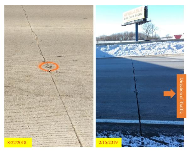
Figure 3.10 Picture Taken from Shoulder of Core #14 Joint on I-41
