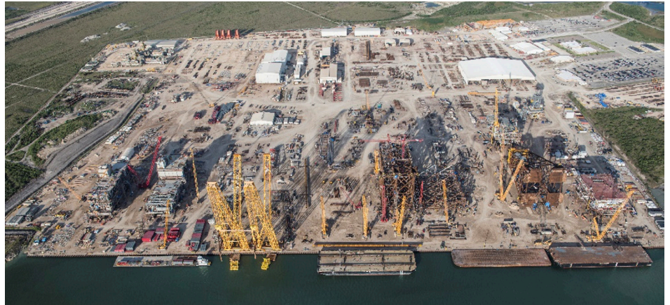
Kiewit Offshore Services aerial overview
