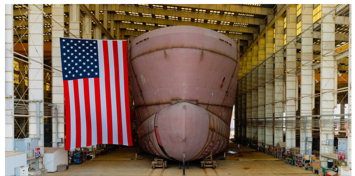
Edison Chouest's Service Operation Vessel (SOV) under construction. Credit: Edison Chouest Offshore Companies
