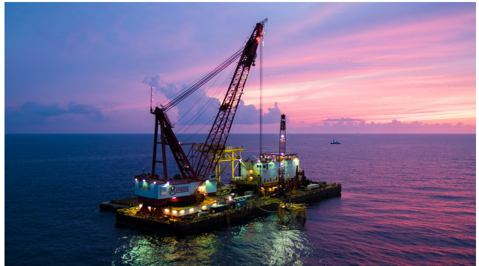
Derrick Barge (Manson Construction)
